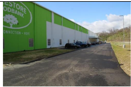
Side of warehouse with pick-up area
