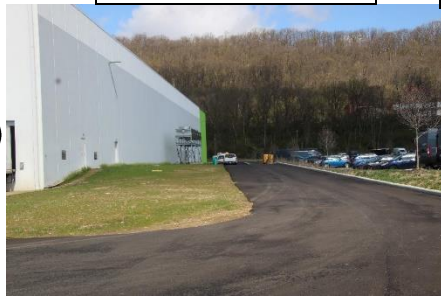
Side of warehouse
