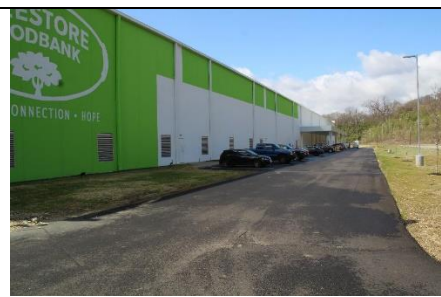
Side of warehouse with pick-up area
